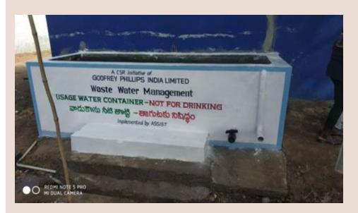
The RO plant while providing safe drinking water also wastes upto 75%. The water with the impurities may leach into the ground. To avoid that the Community RO plants are being fitted with tanks or recharge pits like borewell to keep the ground water intact.
